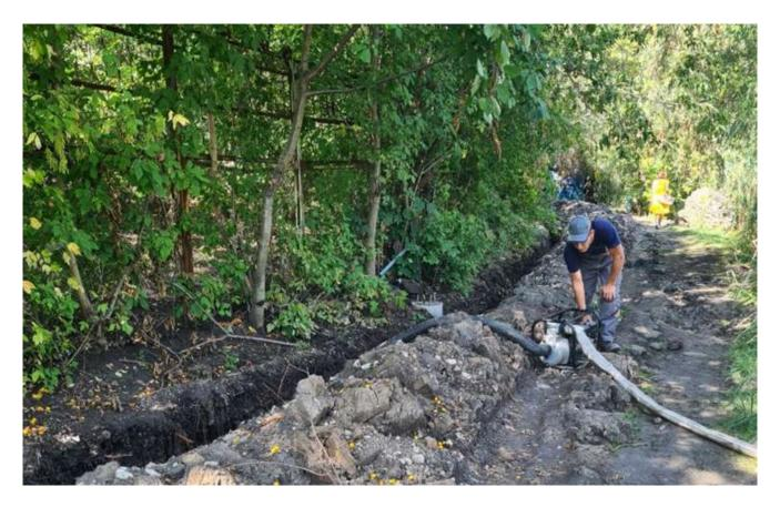
In Vasile Alecsandri Public Garden, the project to install a modern street lighting system has started successfully. The necessary underground works for the electrical power supply network have already been completed, and soon, galvanized metal poles will be installed to host LED lighting sources.
